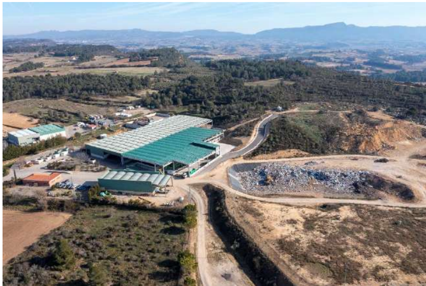
Vista general del Centre
